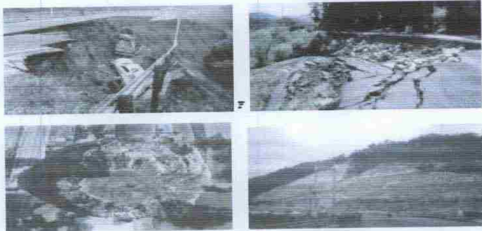
Figure 2-2: Rehabilitation Project Including: (a) Highway Slope Failure Involving Loss of Life; (b) Roadway Landslide; (c) Sinkhole in Orlando, Florida; and (d) Slope Stabilization.
