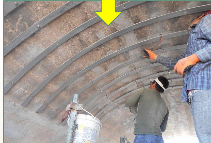
Near Face Reinforcement
