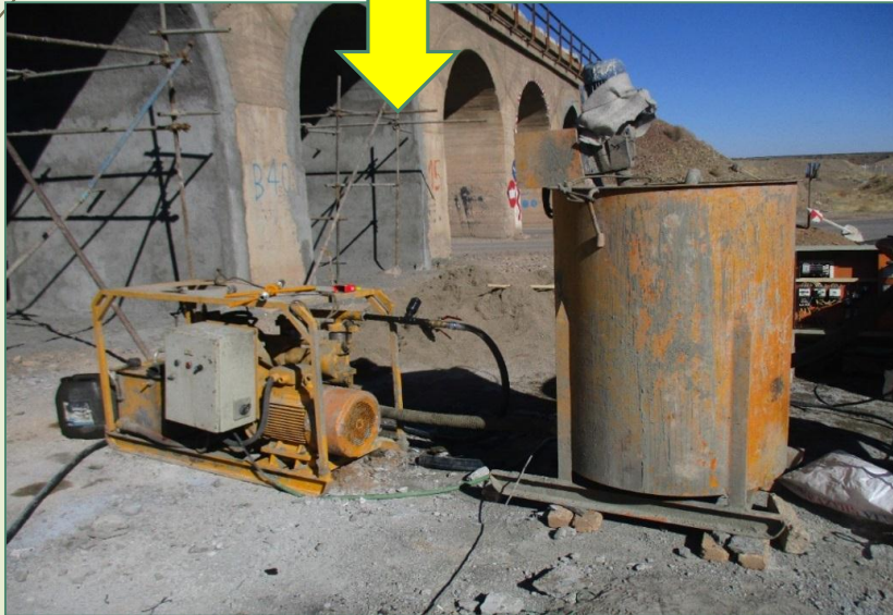
RD Truss Panel + Grout injection
